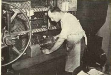
Wheelabrator hubs are an important part of the heart of the Wheelabrator machine. Marion Daxow is performing one of the three inspections on these hubs; testing them on this machine for "run out". The dials show whether the hub is true or not.
